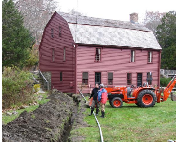
December 2010 trench for burying electrical service in conduit
